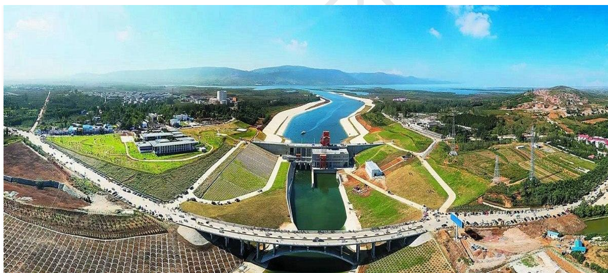
South–North Water Transfer Project Central route starting point taocha in Xichuan County , Nanyang, Henan : Image Courtesy en.wikipedia.org
